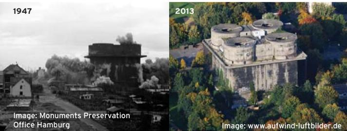
In 1947 the building's interior was blown up by the British army. Six of the building's eight storeys collapsed and the remaining structure became too unsafe for people to enter. The outer shell with up to three metres thick walls and up to four metres thick floors was all that remained relatively undamaged. For over 60 years it was inconceivable that a new use would be found for the whole building, except for some ancillary uses in parts of it.
