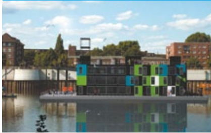
The IBA DOCK Future IBA Hamburg exhibition and office building in the customs harbour
